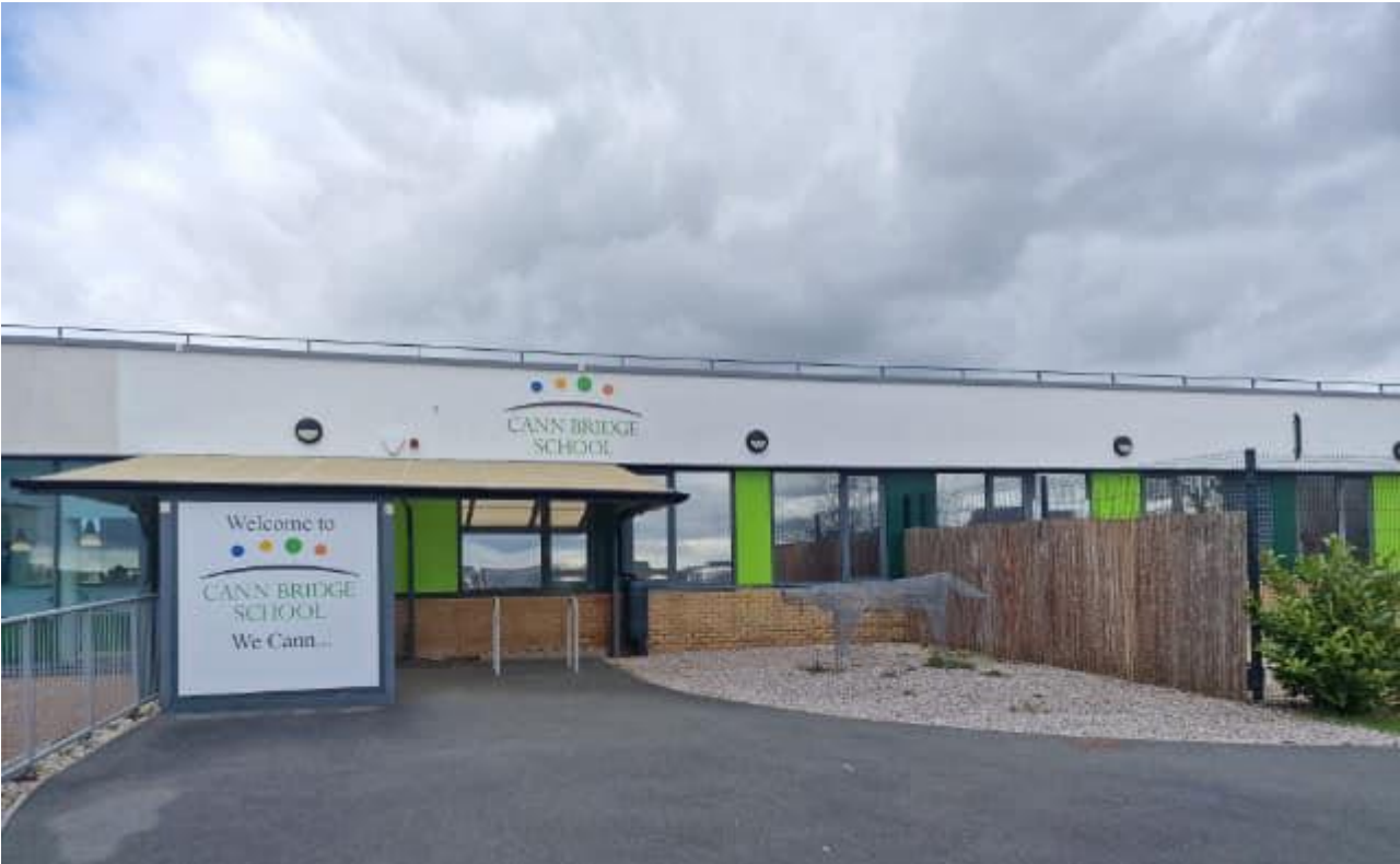
Entrance to Cann Bridge School Reception
